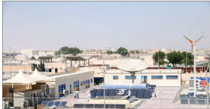
▲ GORD's Technohub, the first novel technology-based platform for research and cutting-edge technologies in the MENA region, aims to assess, develop and promote affordable, clean and efficient solutions. The Technohub consists of a 17.6kW absorption chiller and 25kW desiccant cooling systems driven by a 40kW solar thermal system.
