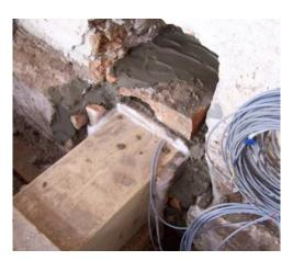
Figure 4. Variant 5 with common halving, aerogel mat around the beam head and as support. Photo: Fraunhofer Institute for Builing Physics IBP.
