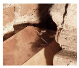
Figure 5. Variant 6 with a copper plate as an artificial thermal bridge. Photo: Fraunhofer Institute for Builing Physics IBP.
