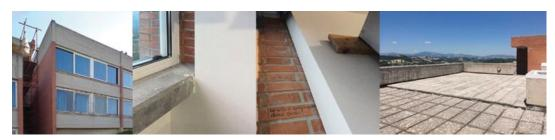
Figure 8. After the pilot site, from left to right: new window, "cold wall" insulation, slab cover.
