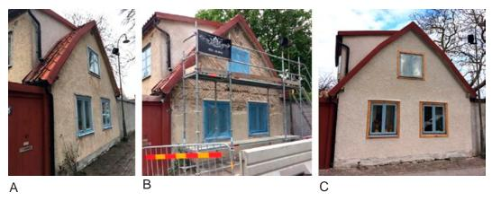
Figure 4. Detached historic single family house in Visby renovated with hemp-lime, A) Before renovation, B) During renovation, C) After renovation. Photos: Paulien Strandberg.
