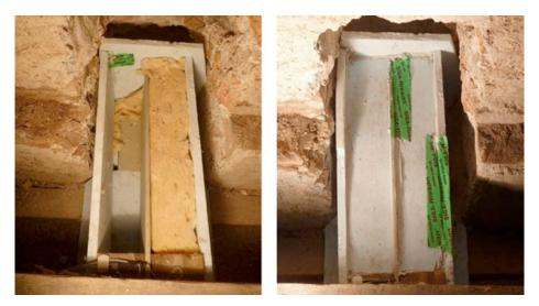
Figure 3. Construction of a box around the metal panel of variant 2, which is filled with mineral wool (left) and then closed (right). Photo: Fraunhofer Institute for Builing Physics IBP.
