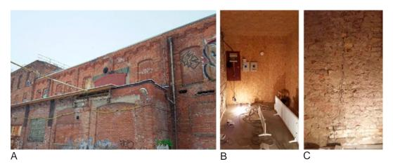
Figure 3. A) Industrial building from 1896 south of Gothenburg to be insulated on the interior with VIP, B) The test room inside the industrial building, C) Sensors in the external brick wall. Photos: Pär Johansson.
