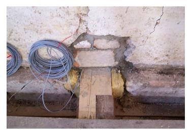
Figure 2. Variant 1 with common halving, mortar bed and insulation mounted around the beam head. Photo: Fraunhofer Institute for Builing Physics IBP.
