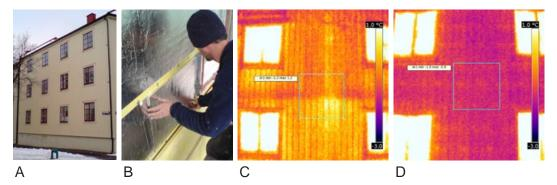
Figure 2. A) Multi-family building from 1930s, B) Installation of VIPs on the exterior, C) Thermography images from 7 February, 2018, non- insulated reference wall, D) VIP insulated wall, average temperature in the square at the intermediate floor between ground floor and first floor is -1.4 °C and -0.2 °C, respectively. Photos: Pär Johansson.
