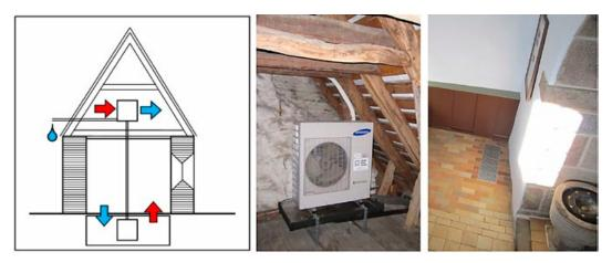
Figure 1. Principal sketch of the heat pump installation in the church (left). To the right a view of the cooling unit in the attic and the inlet in the floor (Erslev Church). Photos: Poul Klenz Larsen.
