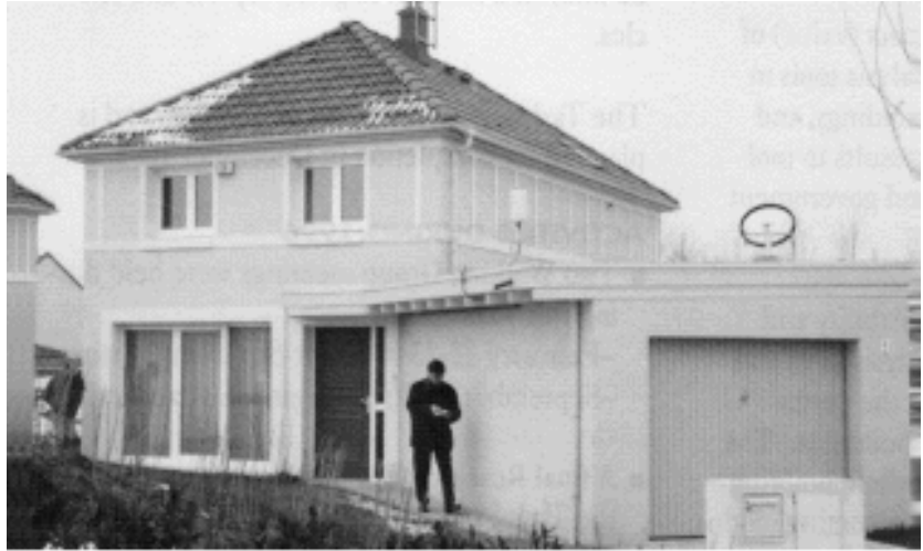
Exterior view of one of the two lisses Test Houses operated by Electricity of France in Lisses, France
