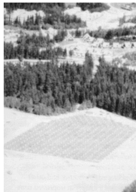
Central solar heating plant with seasonal storage in Lyckebo, Sweden
