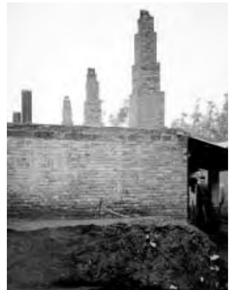
A coal-fired jujube dryer in China
