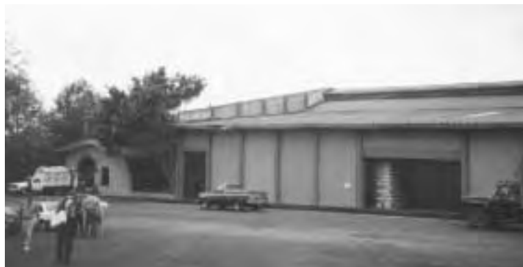
A coffee beneficio in Mexico. The roof is especially adaptive to the installation of solar panels.
