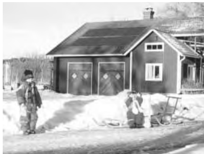
Solar combisystems in Sweden are frequently connected to biomass boilers for back-up.
