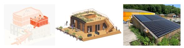
The wood-based building of the VIRTUe team from the Netherlands can be used to add additional floor space to existing buildings. The roof is walkable and includes a PVT field plus a solar collector linked to the house's underfloor heating and cooling system.
