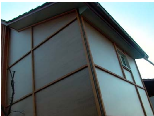
Figure 3.5-48 Façade with the Lucido system applied
