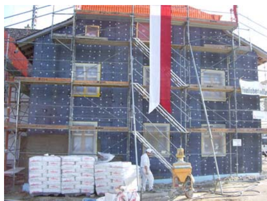
Figure 3.5-44 New exterior wall insulation [114] Source: Agitec. www.agitec.ch/
