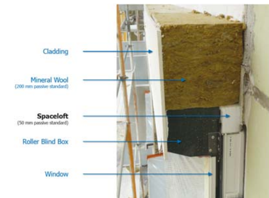
Figure 3.5-47 Insulation of roller blind boxes [118][40]
