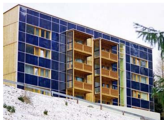
Figure 6.5-8 south façade of an apartment building with 14 flats in Mooserkreuz / Austria. Copyright: Austria Solar [163]
