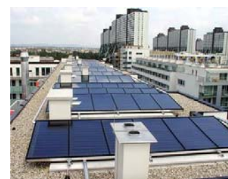
Figure 6.5-1 202 m 2 collector area on a roof of a multifamily building in Vienna (Erlaaerplatz), 200 apartments, 10 m 3 heat store, Copyright: S.O.L.I.D.[192]
