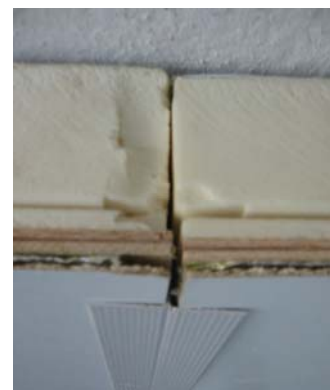
Figure 3.4-1 Realized insulation Tevesstraße. [MHWI 2009]
