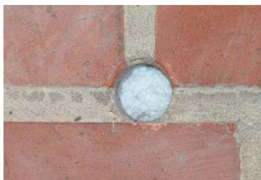
Figure 3.5-30 Opening to introduce the blow-in insulation in the joint area of the facing brickwork. Source: InnoDämm GmbH, www.innodaemm.de
