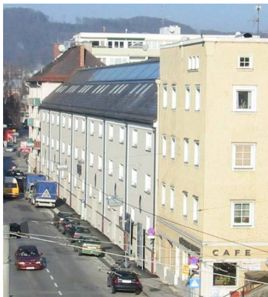
Figure 6.4-11 In the course of a complete modernization a solar thermal system (with 164 m 2 collector area) was installed at the Plainstraße (Salzburg). The non-profit housing company gswb [168] realized there the heat supply concept with a two-pipe system with apartment stations (42 flats).
