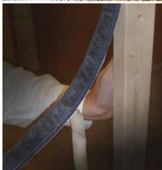
Figure 3.5-41 Retrofitting framing insulation using Spaceloft Insul-Cap [118]
