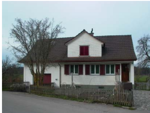
Figure 3.5-52 View of the demonstration building before renovation
