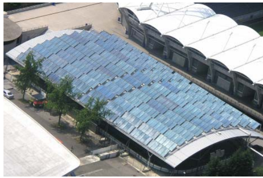
Figure 6.3-2 facilities for feeding-in solar heat in the district heating network of Graz, data source: S.O.L.I.D [192]
