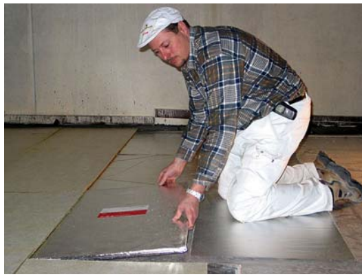
Figure 3.5-12 Laying vacuum insulation panels in the kindergarten
