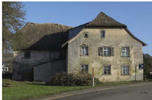
Figure 3.5-42 Existing building before renovation [114] Source: Agitec. www.agitec.ch/
