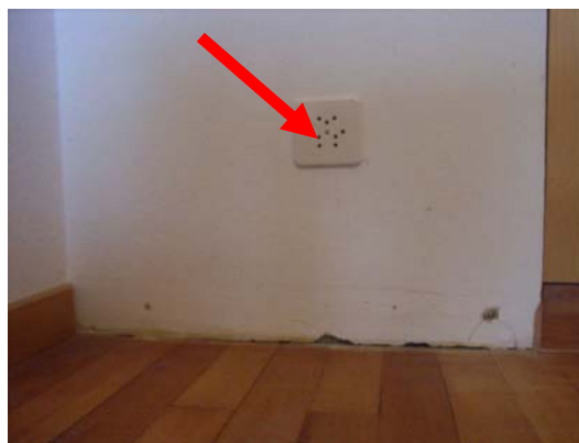
Figure 3.3-3 Inside plaster is not connected to the floor, and the electric plug, covering many air leakage paths.
