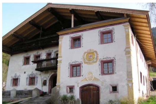
Figure 3.5-5 Thermally renovated listed farmhouse with stone masonry in Kirchbichl / Tyrol
