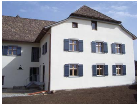
Figure 3.5-46 View of the building after retrofitting [114]
