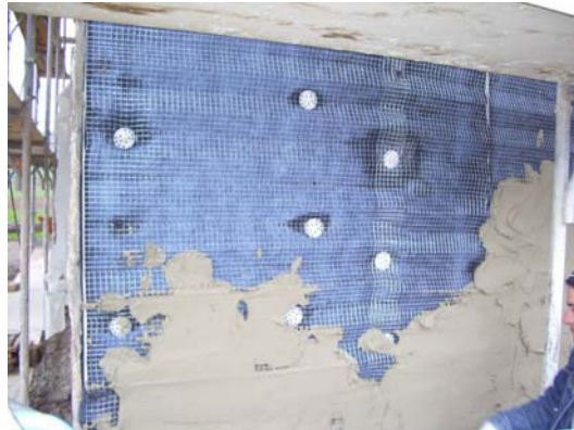
Figure 3.5-45 Fixing and coating of aerogel blankets [114]
