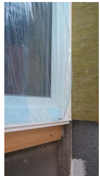
Top and lateral parts should be covered with the exterior wall insulation as far as possible.
