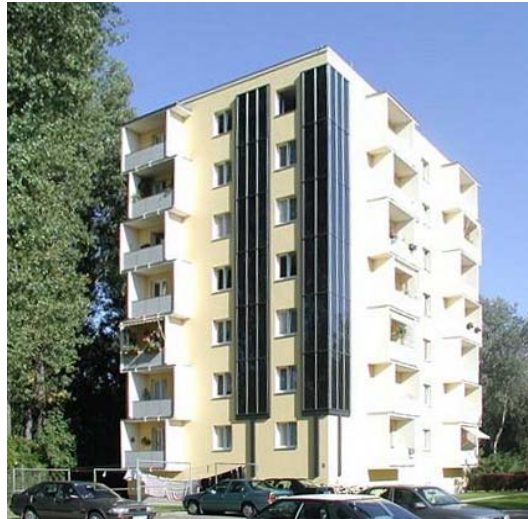
Figure 6.4-5 Striking and well designed integration of 90 m 2 of solar thermal panels into the building façade of the object "Admonterstraße", Krems, image source: GEDESAG [168]
