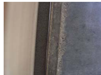
Figure 4.2-25 Craftsmanship is as essential as materials, evidently lacking here.
