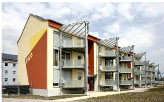
Figure 4.3-1 Renovation project Hoheloogstraße. Left: original building, right: after modernisation in 2006 [Peper/Feist 2009].
