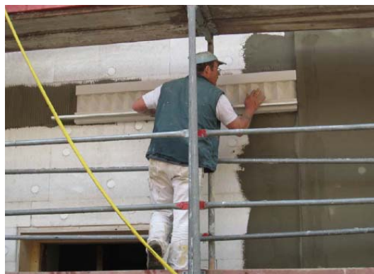
Figure 8.2-8 Placing new cornices over insulation in 142 HIS Purkersdorf AT (Photo: Architekturburo Reinberg)
