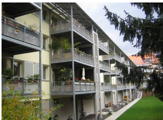
Figure 5.1-1 Demonstration building Blaue Heimat, Heidelberg
