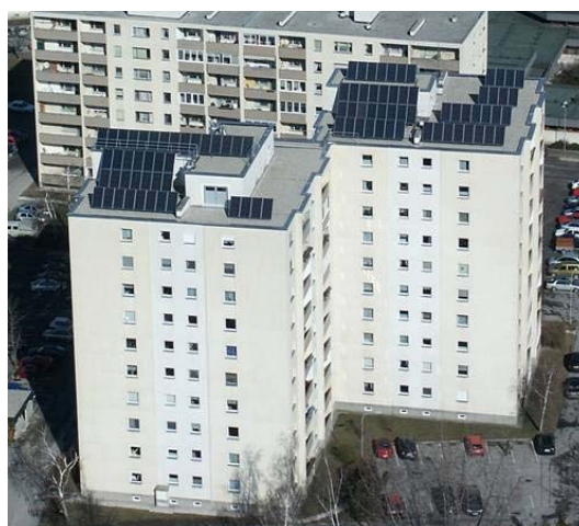
Figure 6.4-7 188 m 2 collector area at the flat roof of the object "Mitterauerstraße" managed by the GEDESAG, Krems, image source: GEDESAG [168]
