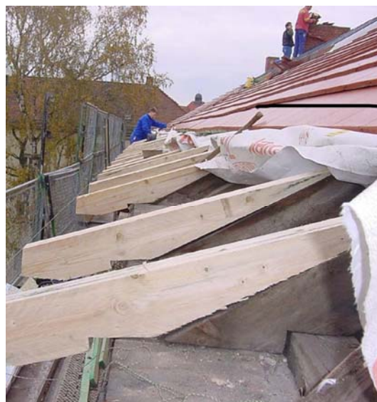
Figure 2.5-7 If the upper ceiling is thermally insulated on top additional parts need to be installed at the roof edge to lift the roof tiles to give room for the insulation layer.
