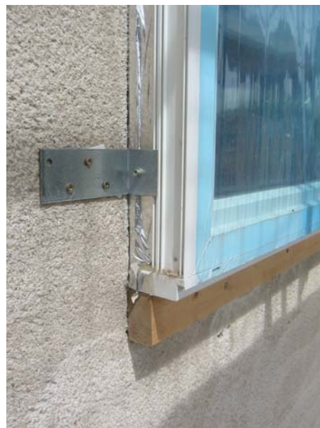
A piece of timber facilitates fixture of windows: It is installed and levelled in advance and later on bears the window's weight. The window is then fixed with stainless steel angles.
