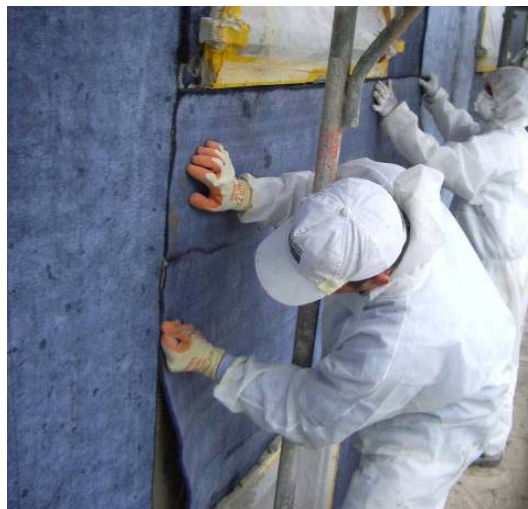
Figure 3.5-43 Mounting Spaceloft aerogel blankets [114] Source: Agitec. www.agitec.ch/
