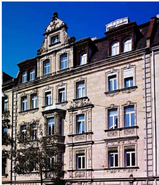
Figure 3.5-4 Apartment house in Fürth near Nuremberg thermally renovated with the new insulation system
