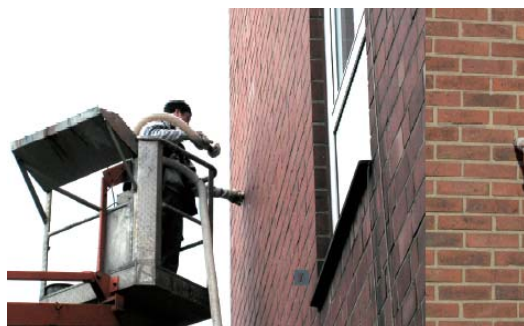
Figure 3.5-29 Backfilling the wall cavity through a hole in the outer shell of the masonry. Source: InnoDämm GmbH, www.innodaemm.de
