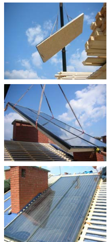
Figure 6.5-7 Mounting of integrated solar collectors on the roof of an attic conversion in Graz, Copyright: Eduard Wasserfaller
