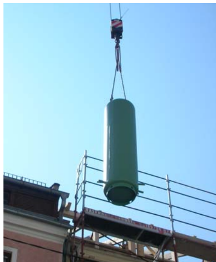
Figure 6.5-9 Example for the emplacement of a standard water store for solar combisystems located in the old town of Graz, Copyright: Eduard Wasserfaller
