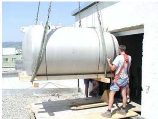
Figure 6.4-6 Altogether 12 m 3 energy storage volume in the heating control centre of the flat roof, image source: GEDESAG [168]
