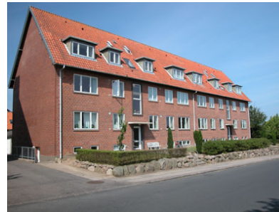
Figure 7.1-16 Existing façade of apartment house in Assens (1930 – 1950).
