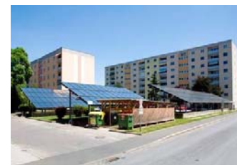
Figure 6.5-2 solar collectors build as outdoor car roofing for an apartment building in Graz (Grottenhofstrasse) Copyright: ENW Ges.m.b.H.
