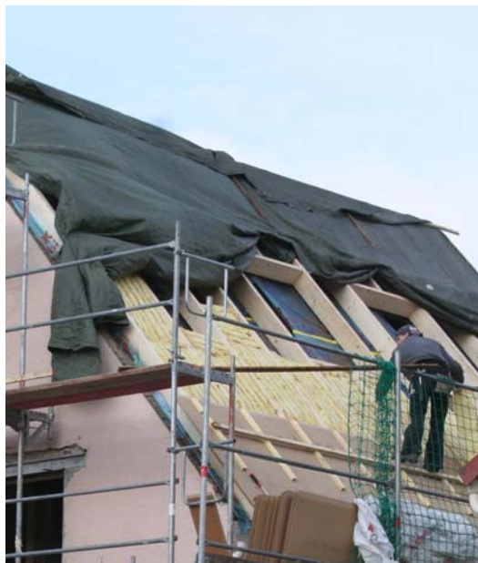
Figure 2.5-1 Well insulated elements of building envelope are important for high thermal comfort in new buildings and old house renovation. Enlarging insulation layer thickness of a sloped roof by doubling the rafters. The gaps are filled with mineral wool. Foto: PHI
