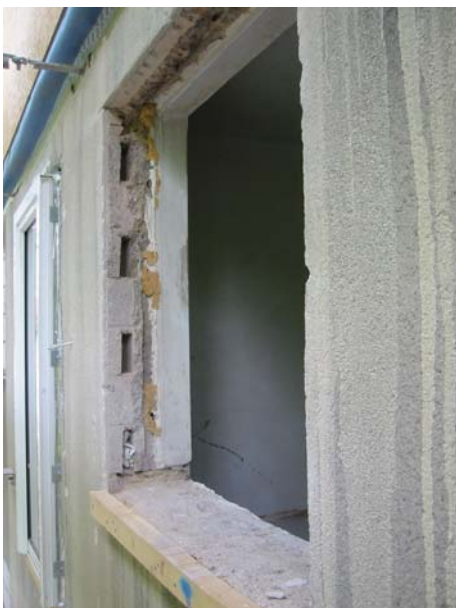
Figure 3.4-39 Window-opening with masonry-rabbets removed
