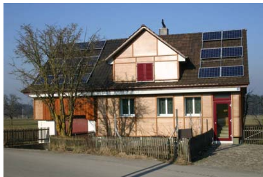
Figure 3.5-53 View of the demonstration building after renovation
