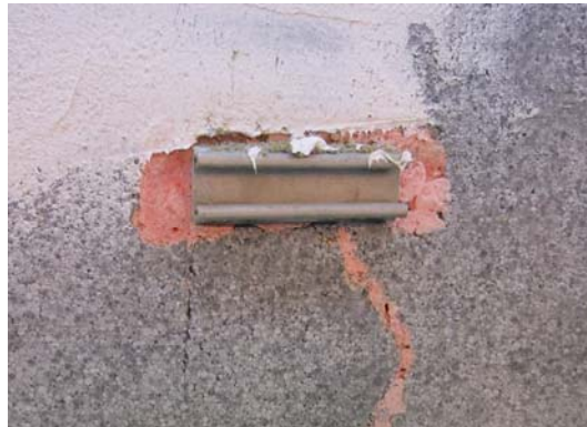
Figure 3.4-46 Stainless balcony tie: anchoring channel on 10mm stainless cantilever bolted through exterior wall with interior conterpiece.
