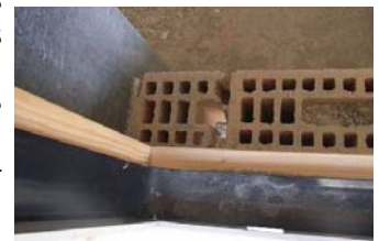
Figure 4.1-1 Leakage near the window frame evidenced by light penetration.
