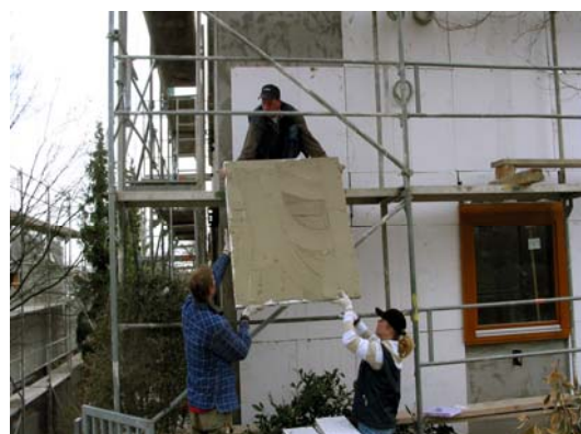
Figure 3.5-21 Covering the vacuum insulation panels with polystyrene panels (left)
