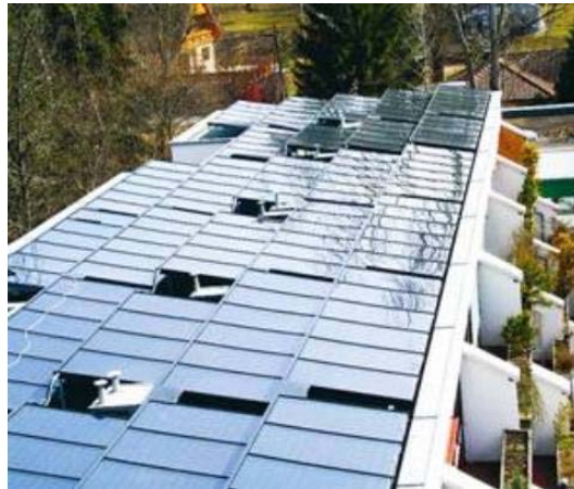
Figure 6.4-8 Afterwards installed solar thermal system (collector area 320 m 2 ) on the flat roof of a housing department in the Hans Riehl Gasse in Graz, supply into the central domestic hot water preparation, image source: [192]
