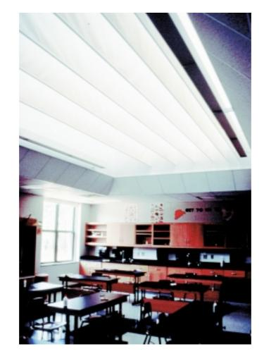
Picture 2 -A typical roof monitor seen from below. This shows the hanging baffles that diffuse the light, creating a more uniform distribution of light and eliminating all beam sunlight that would otherwise cause glare.
