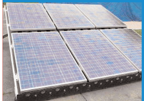
Preparation of the test stand for the air PV/T collector at the National Solar Test Facility in Canada.
