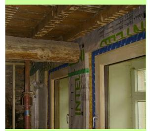
The inside wall insulation and continuous air tightness screen: turning a set back into an advantage
