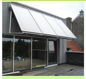
Combination of the solar panels also serving as sun shading for the upper windows.
