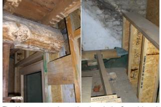
The I-beam construction cutting through the floor slab and support beam (left) and ending above the upper floor level, next to the new roof construction (right). The brick wall clearly shows were the old roof was.
