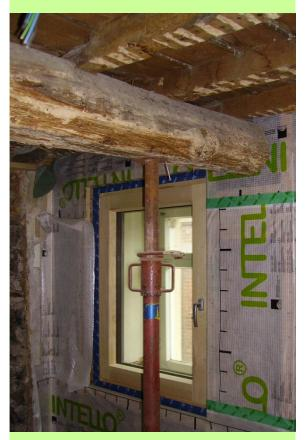
Problem of air tightness on old beam. Note the 'intelligent' air and vapour tightness screen The screen's vapor resistance is varying depending on the relative humidity, going from 0.25m to 10.5m.
