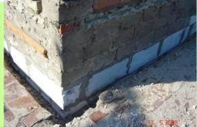
Thermal break at the base of the walls
