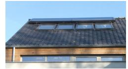
The roof windows and the solar thermal collector.
