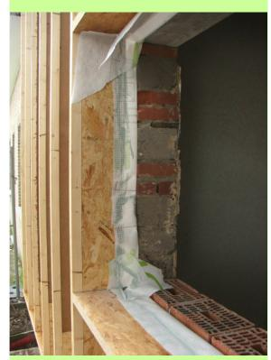
Timber frame construction fixed to the existing wall. The originally wall was erected with concrete blocks, but during the retrofit and the adaptation of the windows some clay tile blocks were build in.
