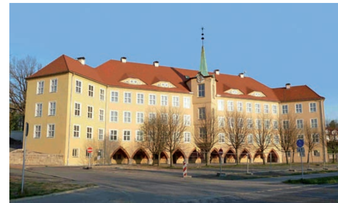
3-litre-school building at Olbersdorf after refurbishment
